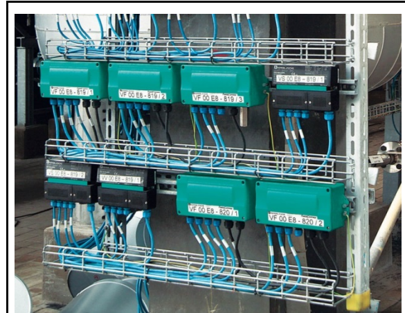
Figure 20: Fieldbus installation in cable trays.
